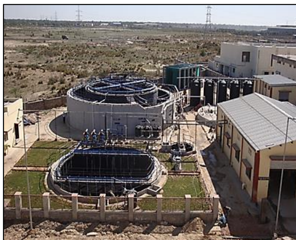
Figure 2: Typical view of the facility
