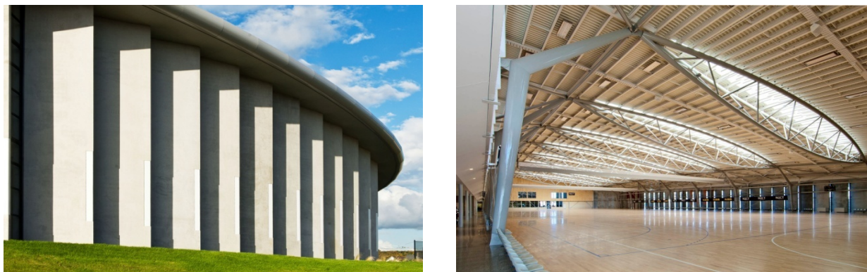
Figure.4 ABS Sports Center use simple and appropriate envelope material according to the local climate characteristics
