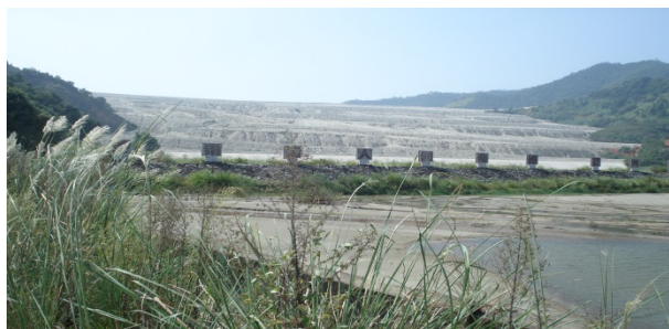
Figure 1 On-site photo of high tailings dam
