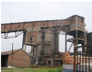
Fig 1: The main structure of belt corridor of ChaCheng coal
