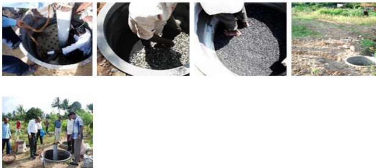
Fig 1: Installation Or Injection Of Bore Well
