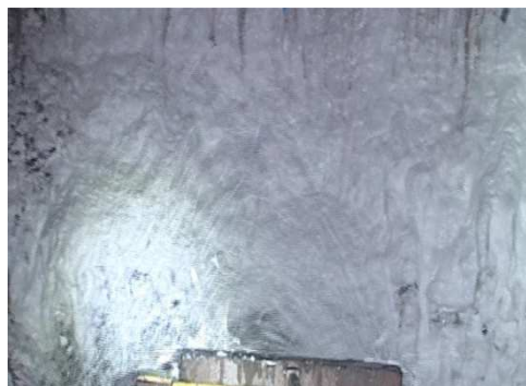
Fig. 13 Suppressing dust by injecting foam
